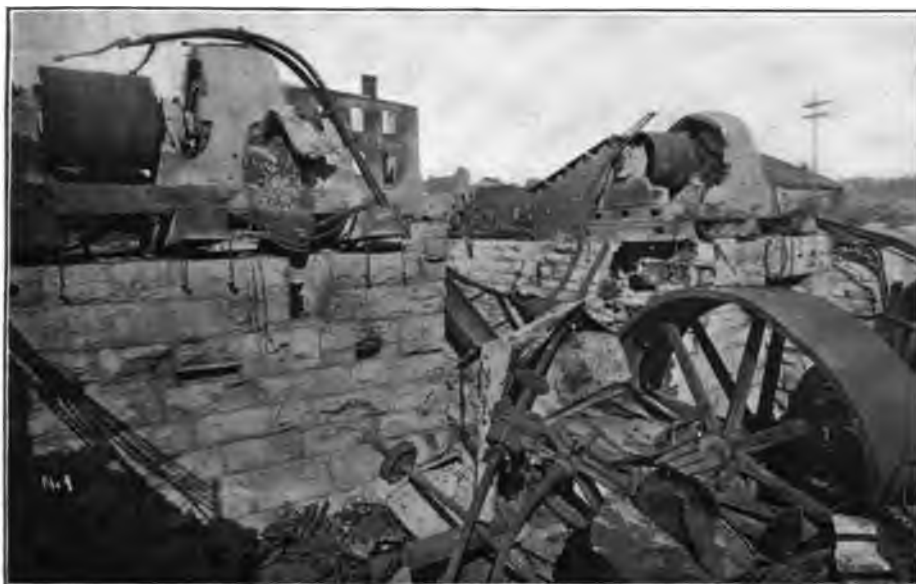
PHOTO. BY PITTAWAY. OTTAWA—THE ELECTRIC CO.'S POWER HOUSE.
